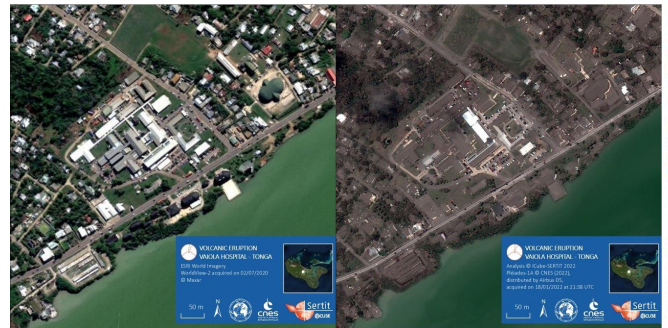
Figure 4. Before and after view of Vaiola Hospital in Nuku'alofa, capital of Tonga.
